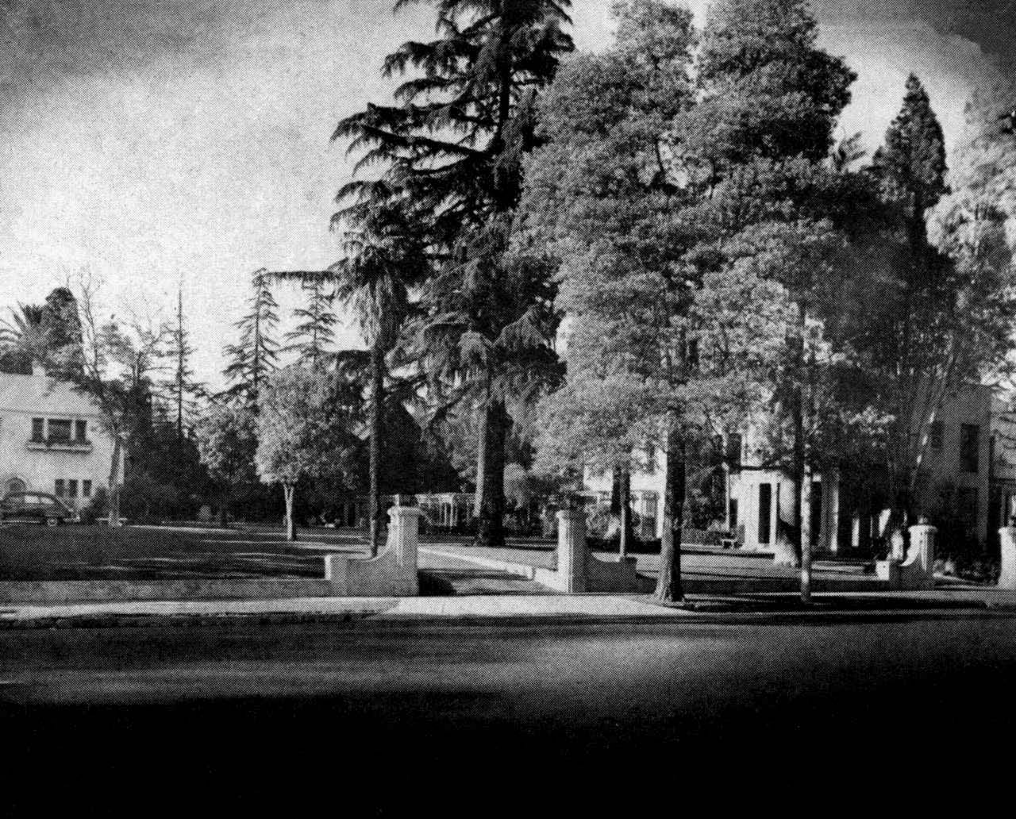
Entrance to Ambassador College. Main building, right, and corner of administration building, left.
